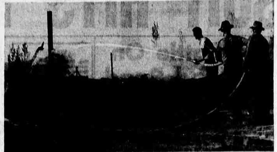
Sparks from a trash fire burning in front of the old Anderson Motor company building late Thursday afternoon, destroyed the structure and brought out city and county fire trucks and volunteer firemen. The building was in the process of being razed by Frank Gabriel, Olene farmer. Property is owned by Swan Lake Moulding company.
