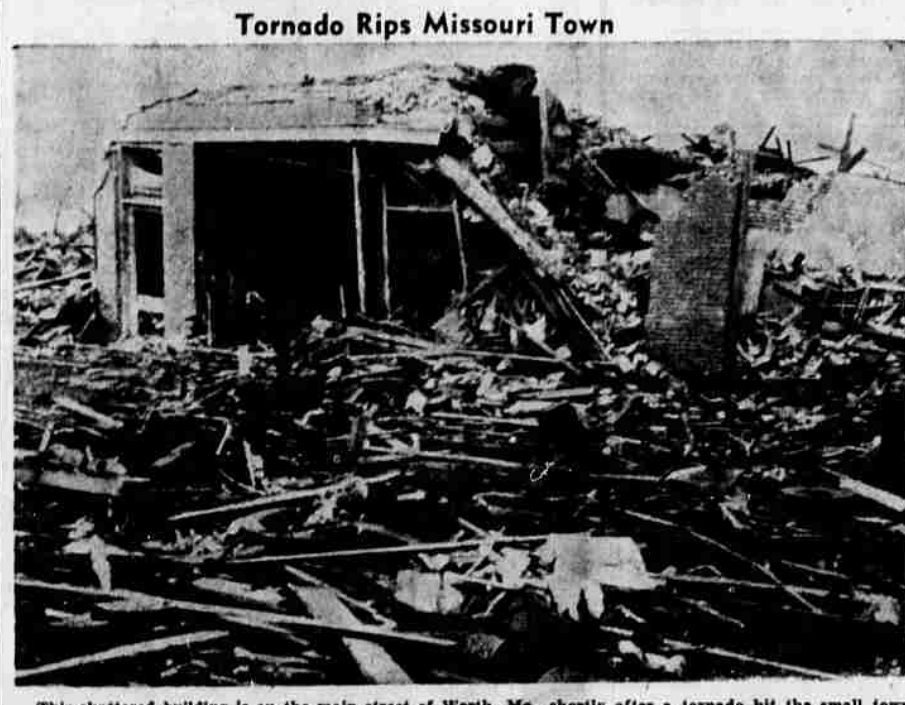
This shattered building is on the main street of Worth, Mo., shortly after a tornado hit the small town. It was near this building, the C. B. Adams feed store, that two men were killed.
