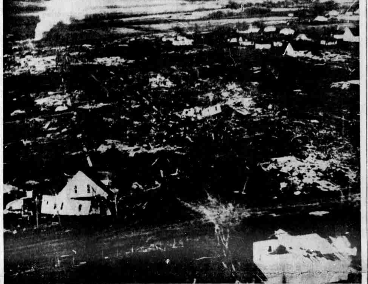
WORTH, Mo., April 30—Its walls pushed apart and its roof collapsed, the house in the foreground was among those damaged by a tornado which tore through Worth, Mo., today.
