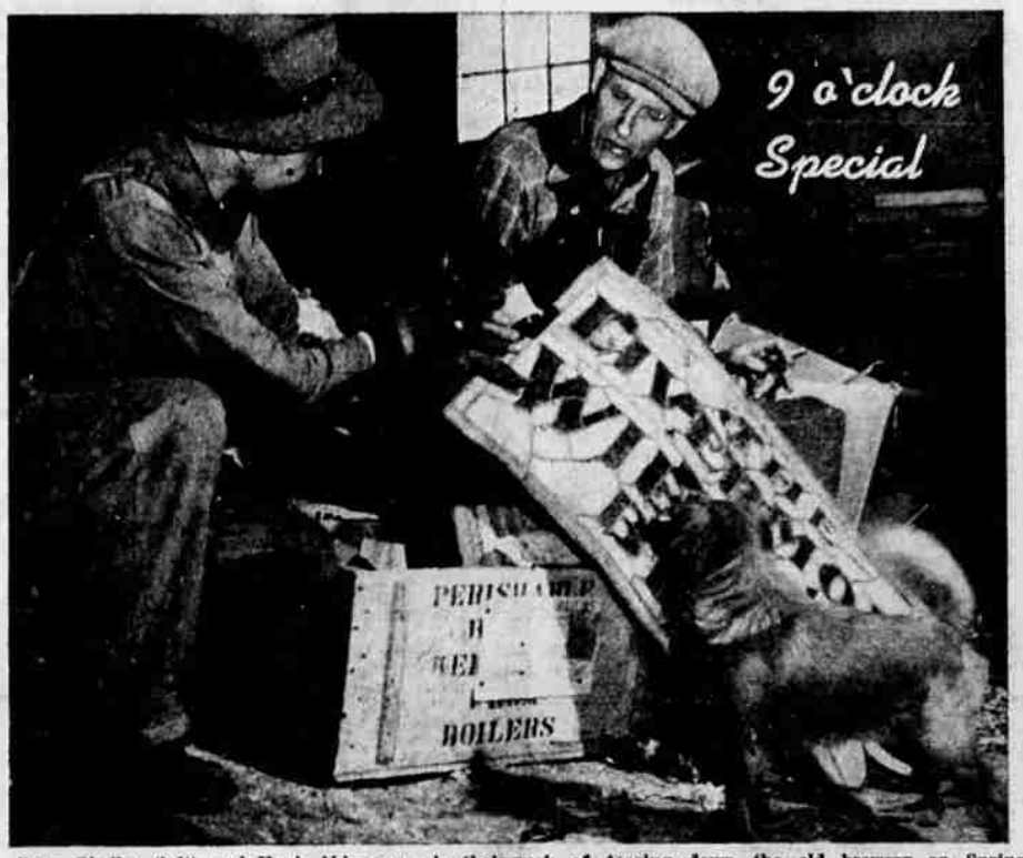
Gene Gheller (left) and Hank Akin pause in their work of tearing down the old brewery on Spring street, to inspect bottle which once held 1900 vintage of Rudesheimer wine. Leaning against a pile of debris is an old stained glass sign advertising the Livermore bar which stood on Main street where Gus Anderson's service station now holds forth.
