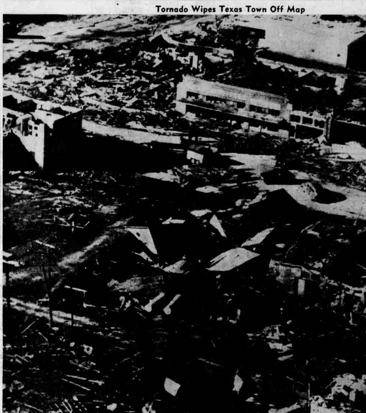
HIGGINS, Tex., April 10 (AP)—This picture, taken from the air, shows the town of Higgins, Tex., after a record breaking tornado swept over it yesterday afternoon demolishing the business section completely. The tornado ripped and slashed across the Panhandle, creating havoc in one of the richest cattle and wheat lands in the nation. This picture was rushed to The Herald and News by AP wirephoto with the aid of local telephone officials despite the crippling telephone strike. —AP wirephoto.
