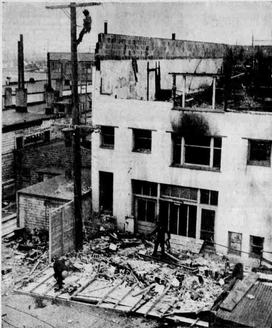
A 47-mile gale ate out a portion of the rear wall of the Evans apartments and sent the east wall weaving and buckling before a large crowd of onlookers at noon today. No one was injured when the top section crashed and occupants of the buildings on Main adjoining the fire-gutted building were evacuated by police and firemen as a safety precaution.
