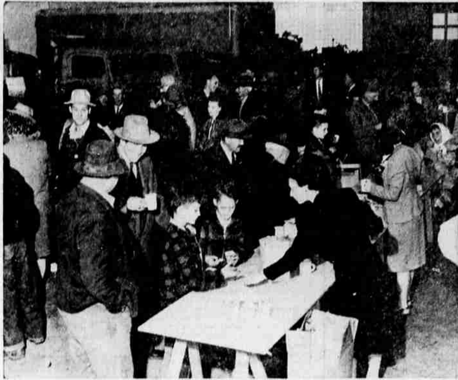
This picture shows a few of the 800 to 1000 people who visited the new West-Hitchcock plant last Saturday. Refreshments were served in the shop, shown above.
