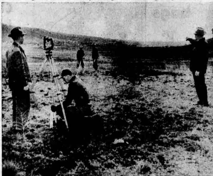
Looking Toward The City Along The New Highway Entrance
