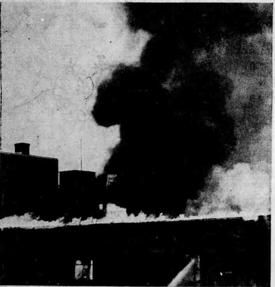
VIEW FROM THE PELICAN HOTEL across Main street, showing the top of the Evans building just as flames completed the destruction of the roof.
