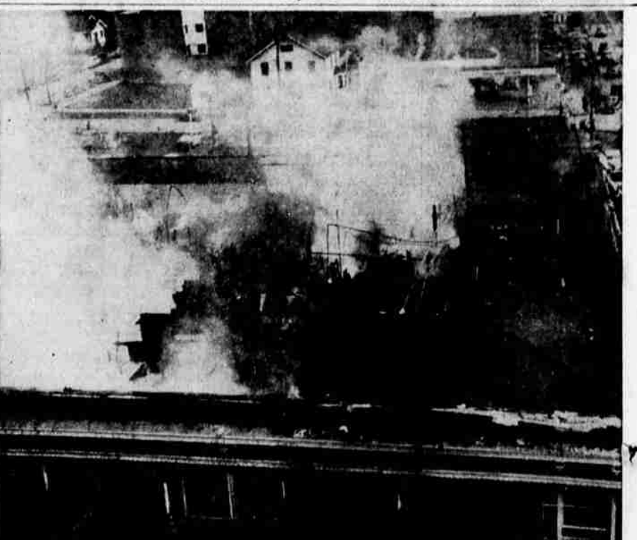
THIS PICTURE, taken about 10:30 a. m., shows the smoking interior of the building as seen from the top of the Medical Dental building across Tenth street.
