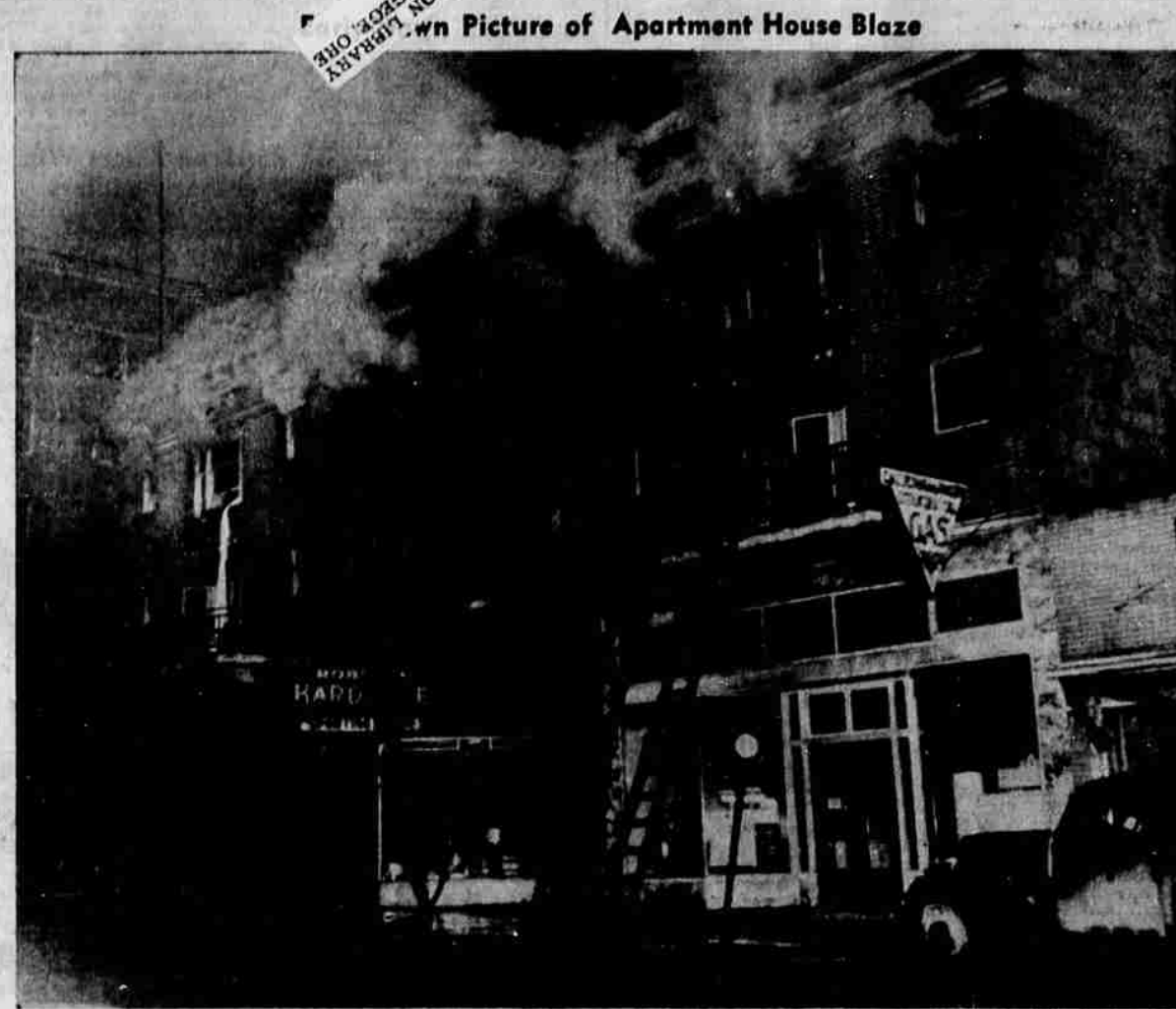
This picture, taken only a few minutes after fire was discovered at Evans apartments, shows the smoke pouring from third-story windows as firemen look through for more survivors. The top story burned before the second floor. Notice the bed sheet rope in the window where Mr. and Mrs. Carl Arthur and daughter descended to a balcony, and the ladders used to bring other occupants to safety.
