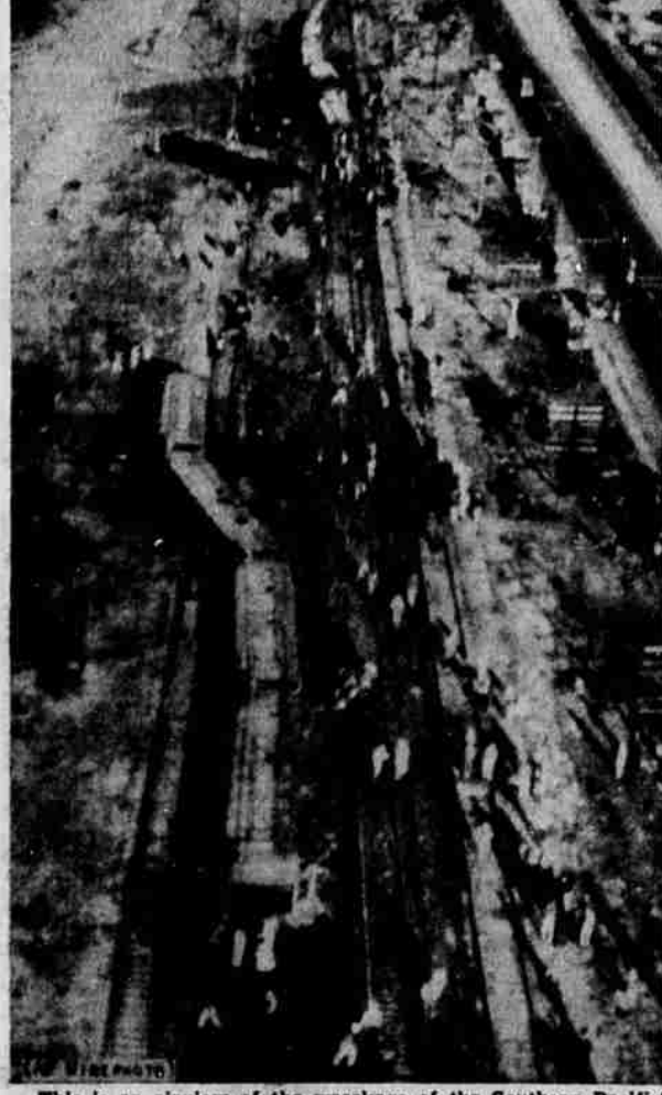
This is an airview of the wreckage of the Southern Pacific's Owl crack night train, six cars of which overturned when the train hit a broken rail near Bakersfield early today. At least seven persons were killed. The picture was received over telephone wire at Klamath Falls before noon today by AP wire-photo service.
