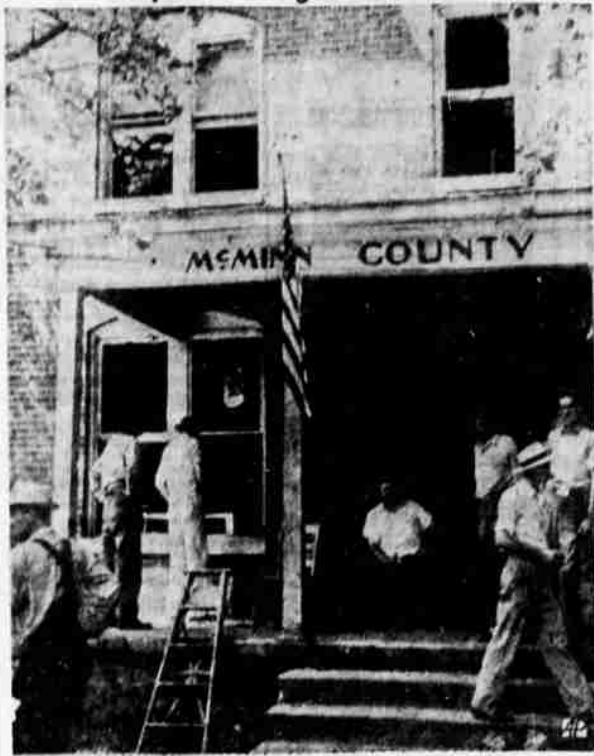
Workmen, under the direction of an interim government, replace windows shot out during a gun battle at Athens, Tenn., between ex-servicemen and the sheriff and his deputies on election day. —AP wirephoto.
