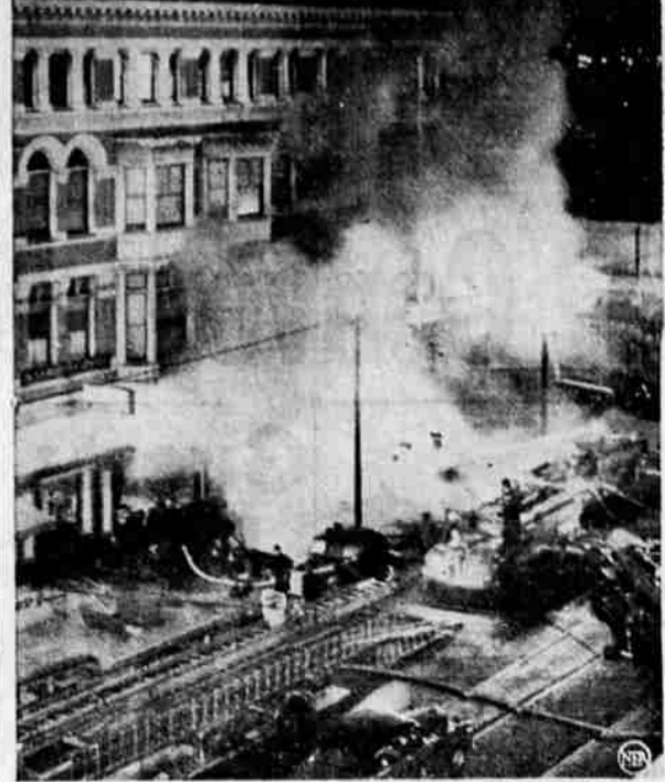
A raging six-alarm fire that gutted Hotel Broadway in Oakland, Calif., was so intense it took 125 firemen 11 hours to subdue the blaze. Twenty firemen were injured in the spectacular blaze that sent pajama-clad hotel residents to the street. The fire caused an estimated $500,000 loss. (NEA Telephoto).
