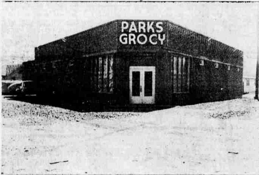
Exterior view of the new Parks Grocery which was constructed by Angelo Doveri, one of Klamath Falls' leading contractors. Plastering on the interior was done by L. C. Ewing, and the cabinet work was done by E. L. Beck. Painting was done by E. A. Smith.
