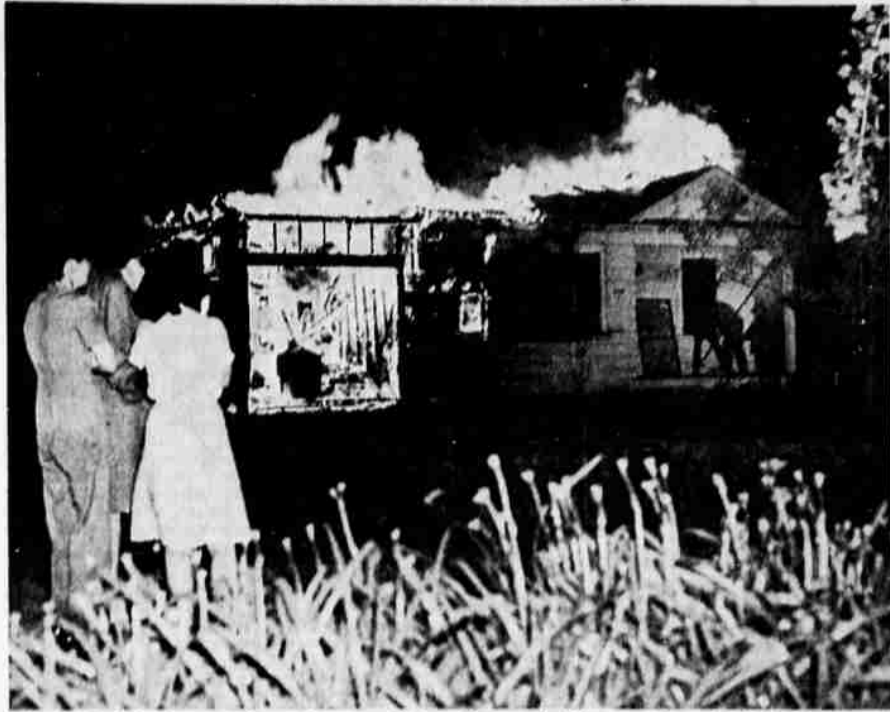
Fire which broke out about 10 p. m. Wednesday resulted in an estimated $9000 damage to a home at 2501 Wiard, owned by J. Reynolds. Living in the house was Bill Davis who was not at home when the fire started. A late fire call was answered by the county fire department. The fire apparently started in an oil storage tank in the garage which adjoined the house, according to the fire department. The house was covered by insurance.
