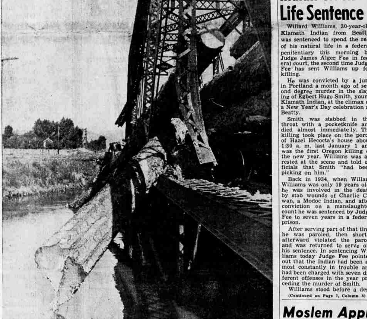
The upper picture shows logs in a twisted mass in the steel bridge at Altamont on the O. C. and E. this morning, after a stake-chain broke and logs on several cars piled up. Below, view along the side of the bridge, showing the damage to the steel superstructure.
