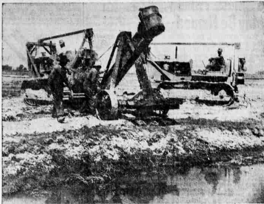
This sub-soiler built by Harold Warner is being used to reclaim 40 acres of basin land which have lain useless since time began. Two large cat-tractors are used with the sub-soiler.
