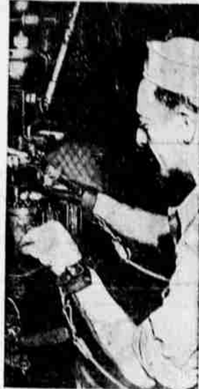
Peter Baker, punch press operator at SKF Industries, Philadelphia, Pa., is literally manacled to his job—and likes it. It's a safety measure which has reduced plant accidents 22 per cent. Shackling device synchronizes movement of the hands with motion of the press. When press descends, cords attached to leather wristbands pull hands out of harm's way if operator doesn't do it quickly enough.
