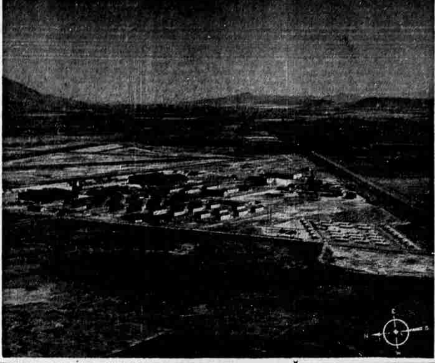
Here are a couple of official navy photographs of the Klamath municipal airport—now a naval air station—which has been the center of local interest and controversy the past fortnight. The upper view looks south, with air station buildings dominating the center of the picture and landing facilities shown at the left, beyond the huge hangars. The lower view looks directly down on the field, giving a graphic view of the runways and taxi strips. The long north-south runway is 7200 feet, the others 5100 feet.
