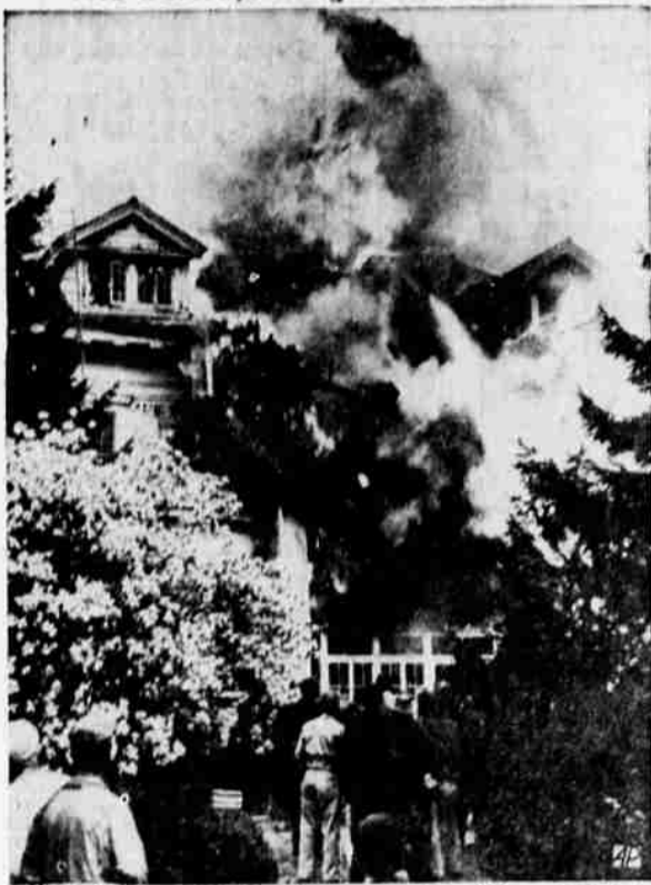
Part of the roof of the 32-room mansion of Samuel Rudel at Roslyn, Long Island, N. Y., caves in as raging flames sweep through the structure. The fire completely destroyed the building and spread to the nearby woods on the estate. Nassau County police estimated the damage at $1,750,000. (AP Wirephoto)
