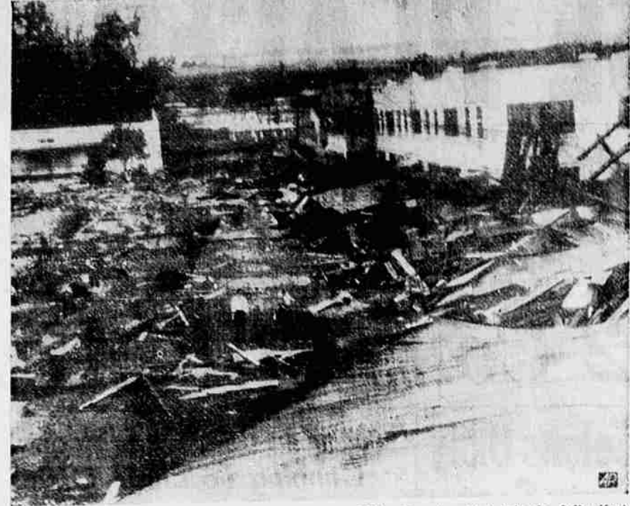
Lumber and debris litters a section of downtown Hilo, Hawaii, which felt the full effect of a tidal wave which hit the Hawaiian islands, Alaska and the California coasts. At least 60 bodies were recovered in Hilo. This picture was transmitted by radio from Honolulu to San Francisco. —AP wirephoto.
