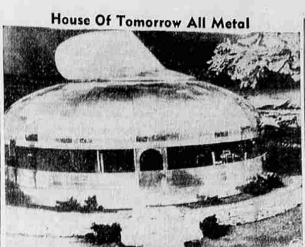
House Of Tomorrow All Metal Promising one answer to the housing shortage is this all-metal, mass-produced Fuller house, which a Wichita, Kas., aircraft firm is ready to produce under license of firm headed by R. Buckmaster Fuller, its inventor. A semi-spherical unit mainly aluminum and weighing only four tons, it can be assembled on site and will sell on ready-to-live basis for about $6500. —NEA telephoto.
