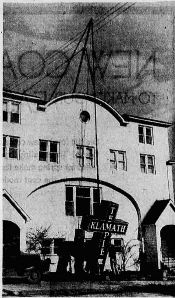
A huge lighted cross was raised to the arch of Klamath Temple, 1007 Pine, this week. The cross, standing better than 12 feet in height, has been erected just above the curved center of the building.
