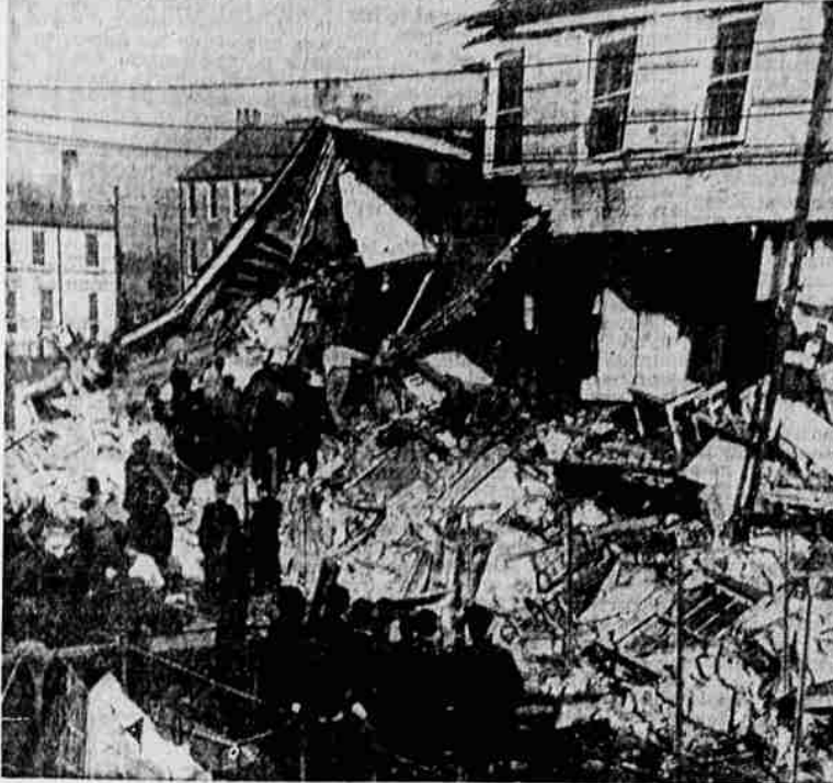
An explosion followed by fire wrecked a three-story apartment building in the downtown residential area of New Orleans, killing an undetermined number of persons and injuring a score of others. Rescue workers are searching through the debris. (AP Wirephoto).
