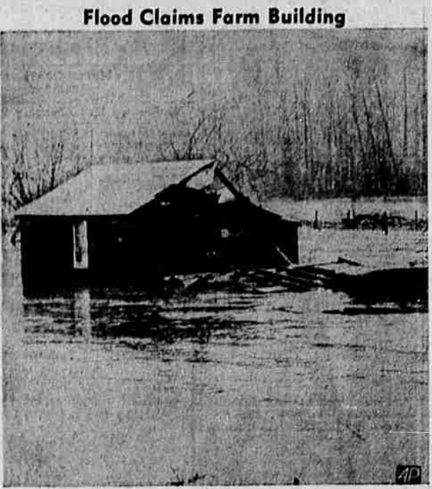
The flooding Willamette river in Oregon is about to wash away this farm building near Springfield in western central Oregon. The top of a parked automobile can be seen at the right of the building. All major highways throughout the western part of the state were closed by slides and floodwaters. (AP wirephoto).
