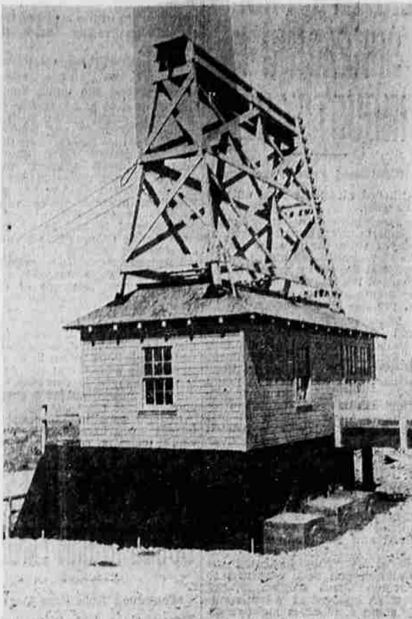
Last of the three scheduled Tule lake pumping plants to be completed is plant "C," located south of the town. It drains an area of 11,500 acres of land.
