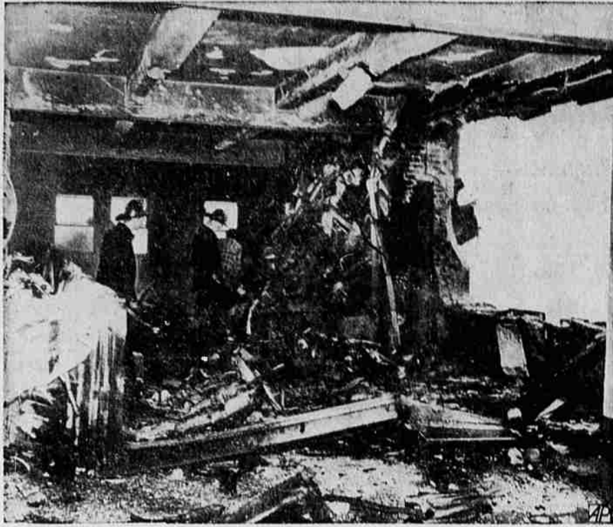
Wheel on the army bomber which crashed into the Empire State building, New York City, is lodged in the elevator shaft. View made from 79th floor looking through shaft to floor below where fireman is looking through debris. (AP Wirephoto).
