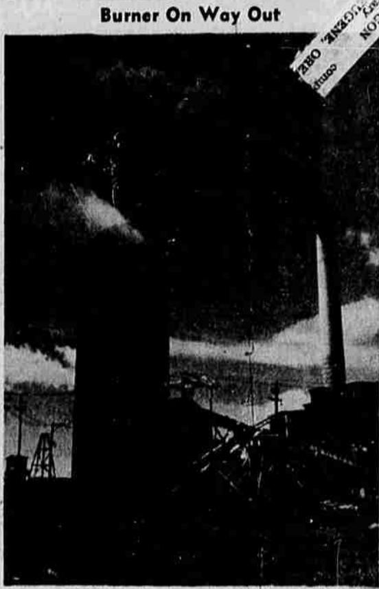
The "For Sale" sign is going up on this burner at the Weyerhaeuser Timber company plant since plans are under way to convert slab and slash waste into chips which will be used for electric power. The passing of the burner marks a change in the lumber industry towards greater utilization of waste.
