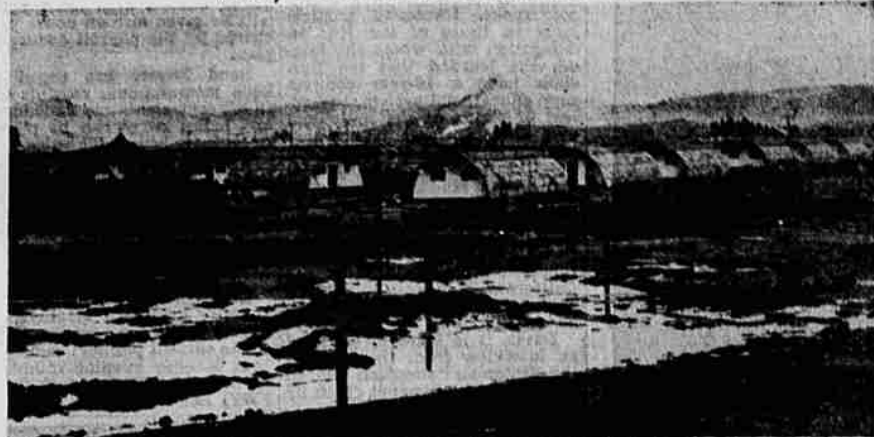
Homaja huts being built to house navy personnel are constructed in the shape of airplane hangars. There will be 31 two-apartment units.
