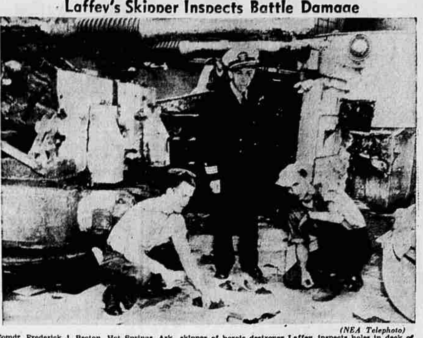
Comdr. Frederick J. Becton, Hot Springs, Ark., skipper of heroic destroyer Laffey, inspects holes in deck of his shattered ship caused by exploding ammunition during terrific battle off Okinawa. With him are TM2/c Derrill W. Stein (left), Kallispell, Mont., and S1/c Raymond T. Johnson, Allentown, Pa. Note the biased gun mount behind them.
