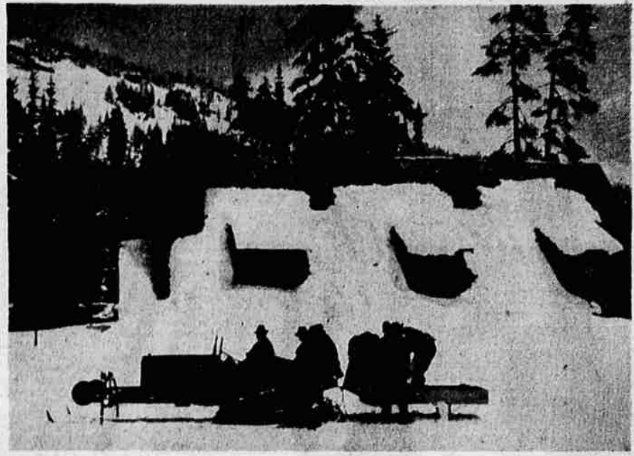
This picture was taken by Assistant Superintendent T. C. Parker of Crater Lake park at park headquarters last weekend, showing a park building and the new snow-traveling vehicle that carried the party into the snowbound interior of the Klamath county recreational and scenic area.
