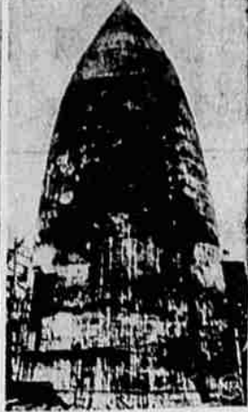
(USAAF photo from NEA) This huge shell-scared, conical structure is an air raid shelter, in which technicians of the Buey-Schloven oil plant, near Gelsenkirchen, Germany, sought protection from Allied aerial attacks which wrecked the plant.
