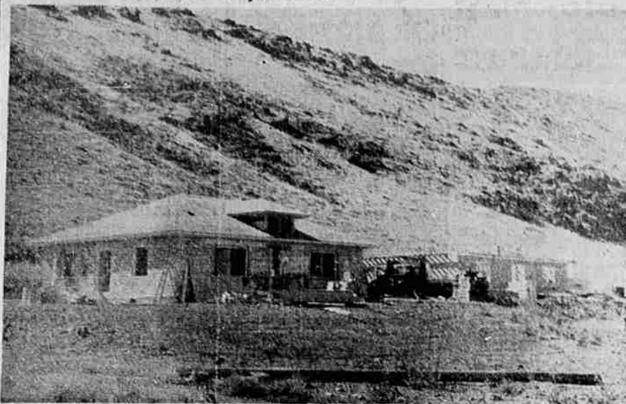
Here are the attractive quarters and other facilities being built for workers for Winema farms, operating a 1200-acre tract on the west side of Tulelake. Steve Takacs, Lee Dixon and Lewis Kandra are partners in Winema farms. The buildings shown above are being constructed of pumice tile, fully insulated, with showers and other conveniences. Especially interesting are the kitchen and dining room facilities.
