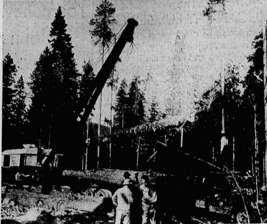
A "jammer" loading trucks at Big Lakes operation near Fort Klamath.
