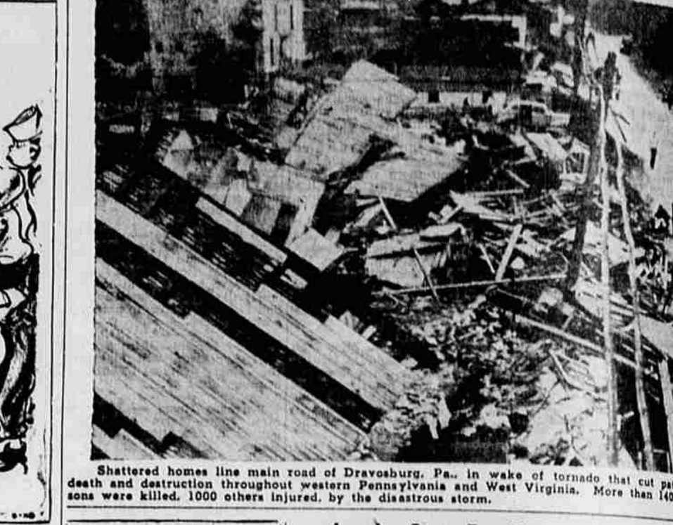
Shattered homes line main road of Dravosburg, Pa., in wake of tornado that cut path of death and destruction throughout western Pennsylvania and West Virginia.
