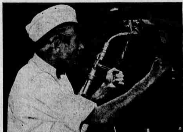
Thoroughness is key of Standard lubrication. Here, shackle is pried for better penetration of lubricant that cuts wear—saves repairs.
