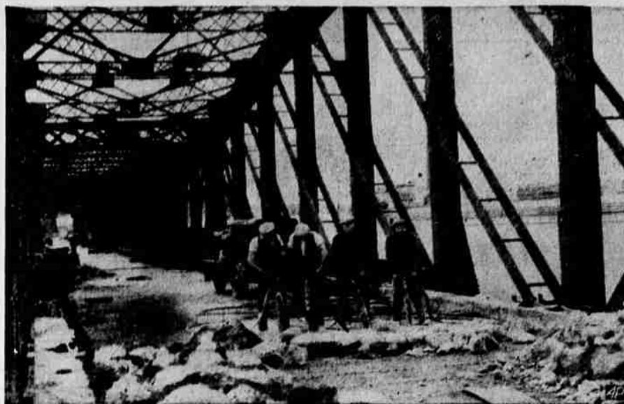
BRIDGE STEEL FOR WAR —London workmen dismantle the "temporary" Waterloo bridge, used for 17 years, to obtain 3,000 tons of steel for munitions.
