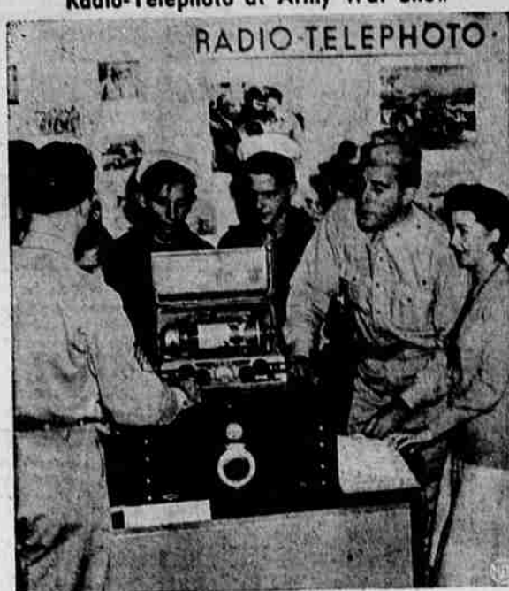
A feature of the Army's Back the Attack-Third War Loan war show in Washington is this display of Signal Corps radio-telephoto equipment, used to transmit pictures, maps and military documents from the war fronts. The Army now uses this equipment, built by Acme Newsictures, to link Algiers and Australia with the U. S.
