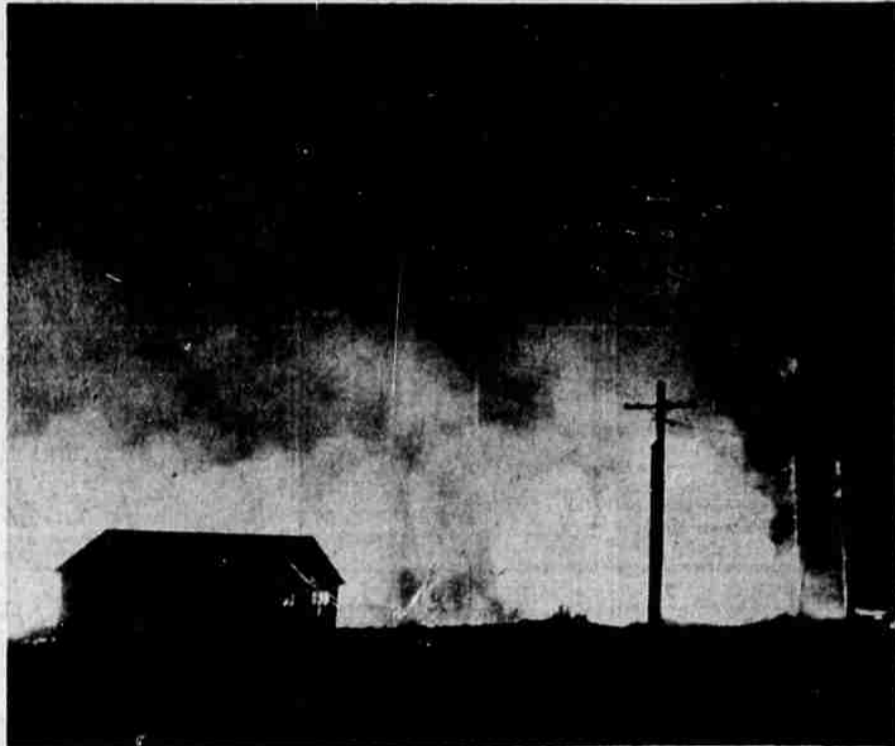
This picture shows the spectacular fire that leveled the old Shaw-Bertram mill buildings on Klamath river Thursday night. The dark building, at left, was saved, but the power tower in the right of the picture finally fell. The buildings belonged to John D. O'Connor, Klamath stockman. The Shaw-Bertram plant was finished in 1923, and operated by Shaw-Bertram and J. Royal Shaw until 1931. In the middle 'thirties it was taken over by Long-Bell, and operated until about a year ago, when it was bought by Weyerhaeuser Timber company. This company dismantled the mill and sold the site to O'Connor for a stock-feeding operation.
