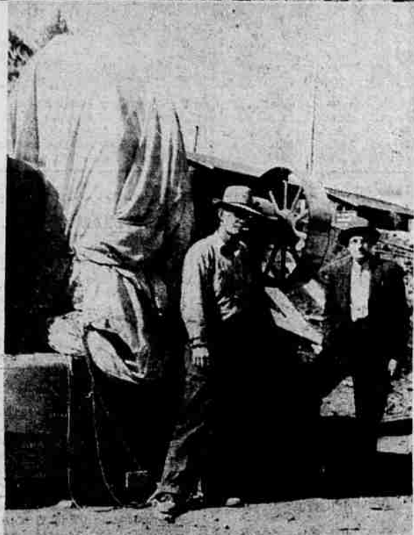
Above, concrete turbine structure of unit No. 2 of the Keno power plant, known as the old Keno plant. The new generator, shown at left, is awaiting emplacement. Men in the picture are K. E. Hutchinson, division accountant, left, and Sam Ritchey, right, division manager. The old wooden superstructure above will be removed. Lower picture: L. W. (Sharkey) Hutchinson, superintendent in charge of the job, and Oscar H. Brennehan, Copco's plant superintendent.
