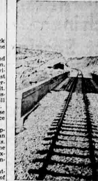
All's quiet at once-embattled Kasserine Pass in Tunisia, where Army engineers have built this new railroad bridge.
