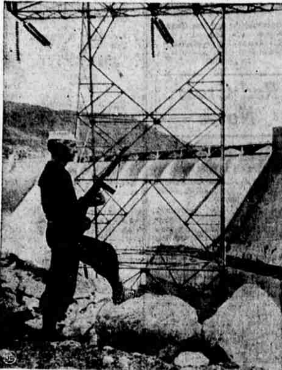
From an elevated post a U. S. coastguardman stands guard over roaring Grand Coulee Dam in Washington. High tension tower is symbolic of electric power generated here for Pacific Northwest war industries.
