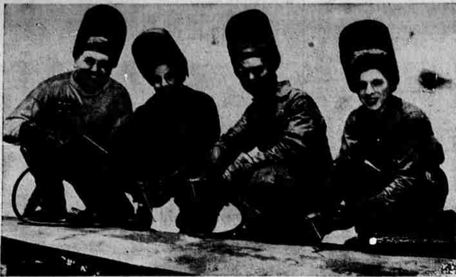
SHIPBUILDING COUPLES — Mr. and Mrs. Michael Kole and Mr. and Mrs. T. W. Fitzsimmons (l. to r.) help weld destroyer escort ships at the Federal shipyard, Port Newark, N. J.
