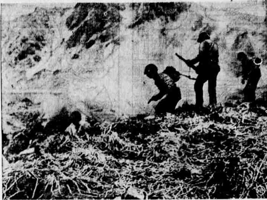
Two Jap soldiers were entrenched in this gun emplacement on the west arm of Holtz Bay when U. S. soldiers staged their recent invasion of Attu Island. Even grenades failed to dislodge them. However, when the Nips, speaking English, dared the Yanks to come and get them, the Doughboys immediately obliged by mopping in and mopping up. Pictured here is the mopping-up process.
