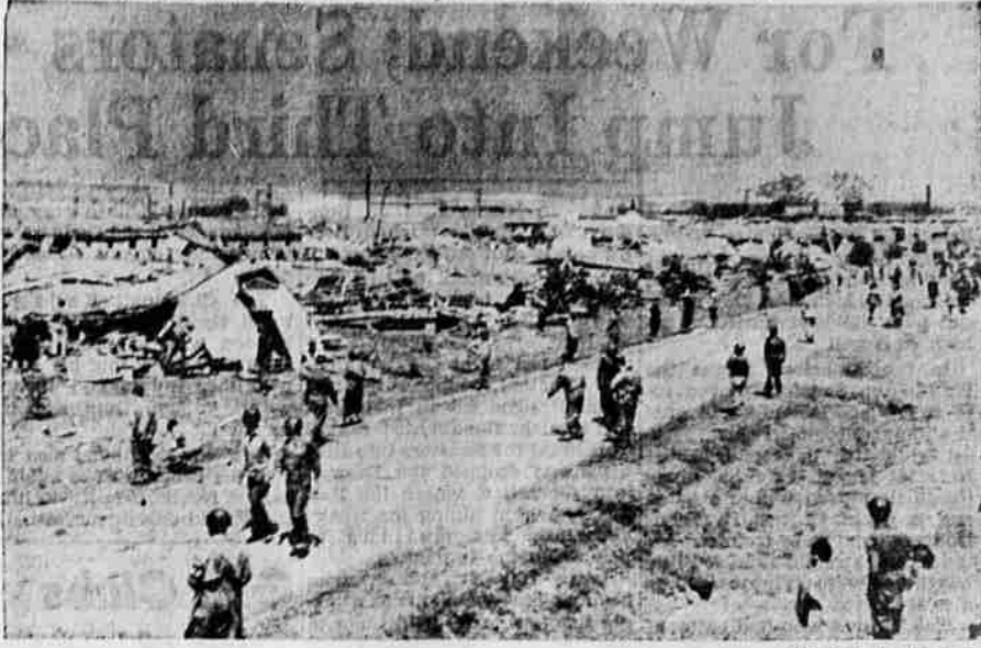
This is what remained of the Fort Riley, Kans., Cavalry Replacement Center after a tornado swept through it on May 15. Forty-seven buildings were damaged, 21 completely destroyed and damage estimated at $178,500. One hundred seventy persons were injured, of which 33 were hospitalized. Photo from Fort Riley Cavalry Replacement Training Center.
