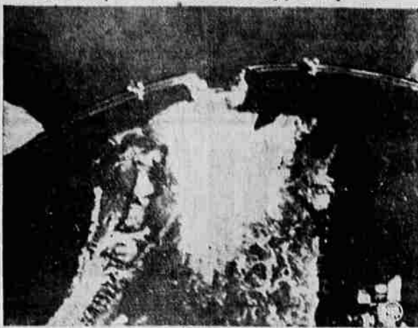
Due to skillful bombing by British fliers, the Ruhr valley, Germany's most important industrial center, had more supply than demand—as far as water was concerned after the RAF's four-motored bombers dropped mines on Mohne dam, causing the breach, shown above, and crippling many of the reich's war industries. Eder dam was also knocked out, flooding the valley and causing heavy damage, which even the Germans admitted.
