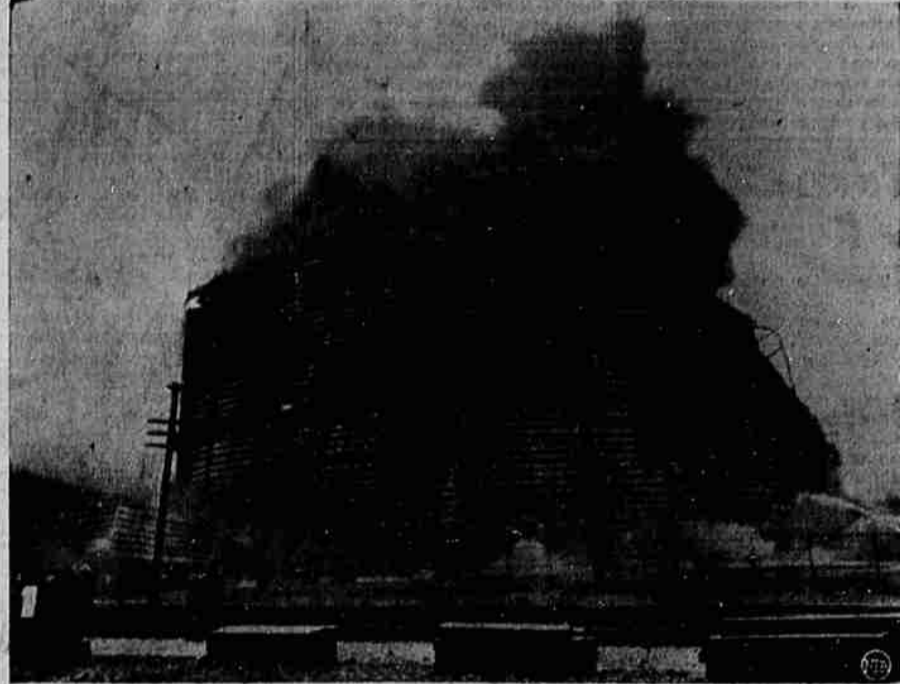
A four-motored army Liberator, flying low and blind through unfavorable weather, plunged into a 150-foot illuminating gas tank two miles from Chicago's municipal airport, turning plane and tank, above, into a seething mass of flames. One charred body and a flaming parachute fell outside the tank, but the remaining members of the 12-man crew burned to death at the bottom of the tank as 18 million cubic feet of gas went up with a roar.
