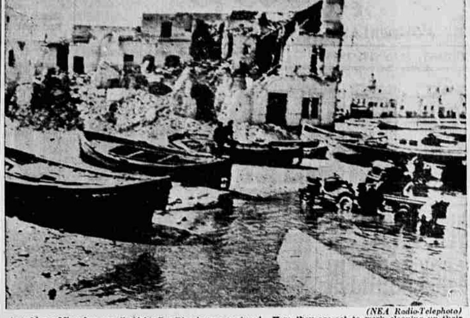
American soldiers keep on the job after Bizerte was captured. Here they are set to work cleaning up their 'jeeps' and 'small trailers' in Bizerte's waterfront. Allied planes inflicted the damage to the building shown in rear, but only 20 casualties were reported due to the expert bombing of Allied flyers. Official U. S. Army Signal Corps, radio-telephoto from Arme.
