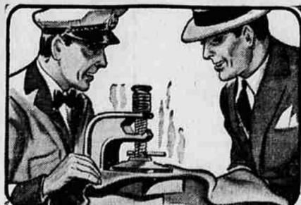
**WE REPAIR BIG RIPS IN TUBES** as well as small punctures. The torn parts of the tube are carefully patched together, vulcanized and then tested for possible leaks. Even torn or leaking valve stems can be replaced. If one of your tires is leaking air, let us examine it.
