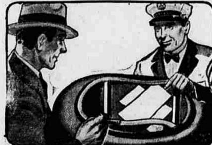
**WE FIX LARGE BREAKS...** First we inspect the tire. Then we clean the injury much the same as a dentist cleans a tooth. A patch is carefully applied, replacing all broken cords. The outside is plugged and the repair is then vulcanized or bonded to the rest of the tire.
