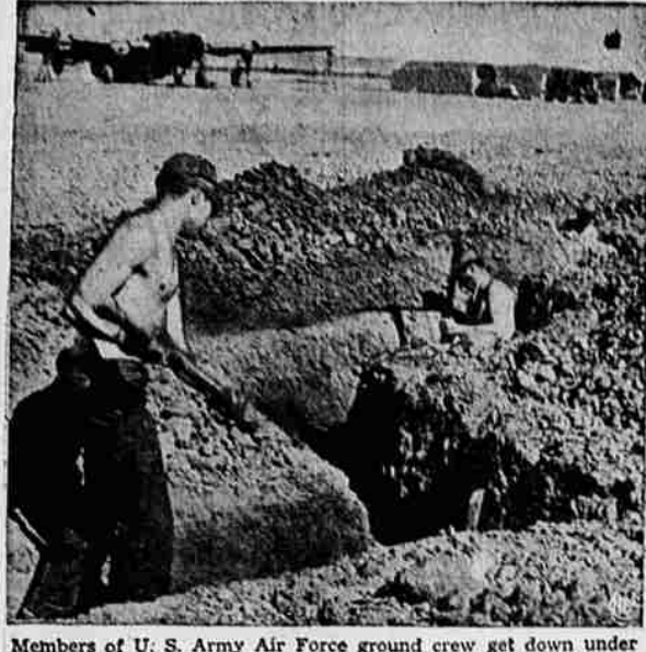
Members of U. S. Army Air Force ground crew get down under the ground with pick and shovel as they dig slit trenches at an airfield in Tunisia. Ditches are used to dodge bombs and to drain the field when it rains. Note big warbird in background.
